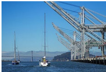
APL Container Cranes Port of Oakland, Oakland CA
