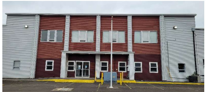
422 Gateway Building exterior
