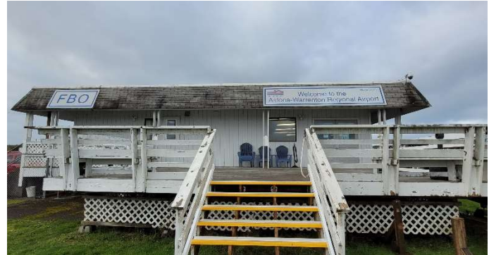
Terminal/FBO Building at the Airport
