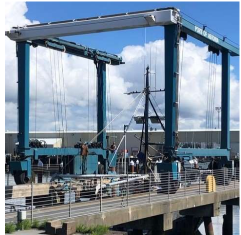
Boat Lift at the Pier 3 Boatyard
