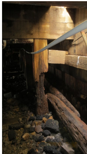
Deteriorated piling under Pier 2 (left) and metal sheets covering the pier surface.
