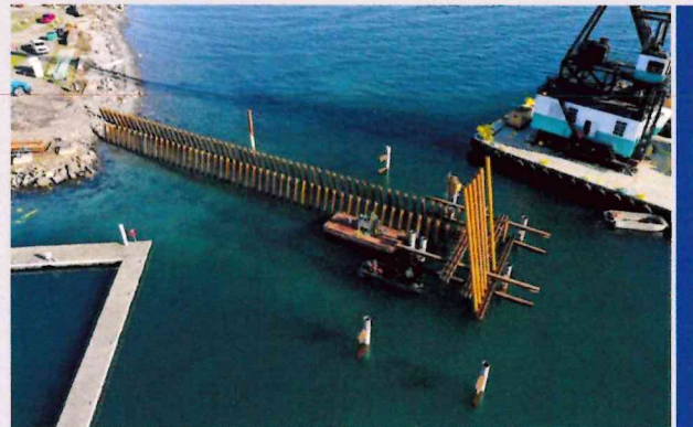
■ Point Hudson Breakwater, Port Townsend Currently under contract
