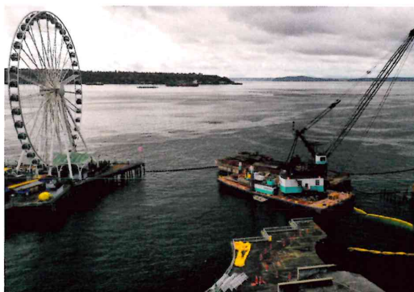
■ Pier 58 Emergency Demolition & Removal Completed 2021
