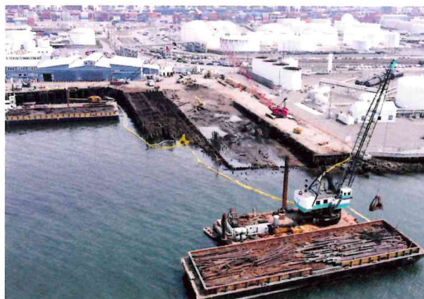
■ Timber Structure Removal - Vigor Shipyards Currently under contract
