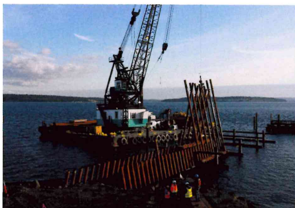
■ Point Hudson Breakwater Installation - Port of Port Townsend Currently under contract
