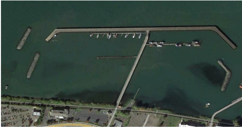
FIGURE 7-1: AERIAL VIEW OF EAST MOORING BASIN
