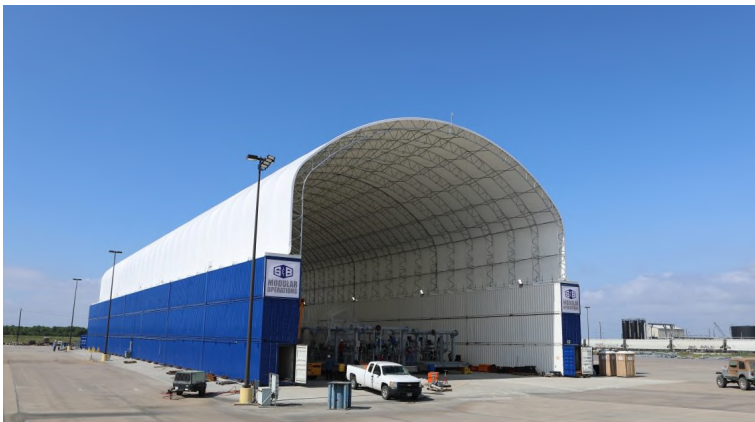
Texas - Module fabrication company serving the oil and gas industries (c/o Big Top Manufacturing)
