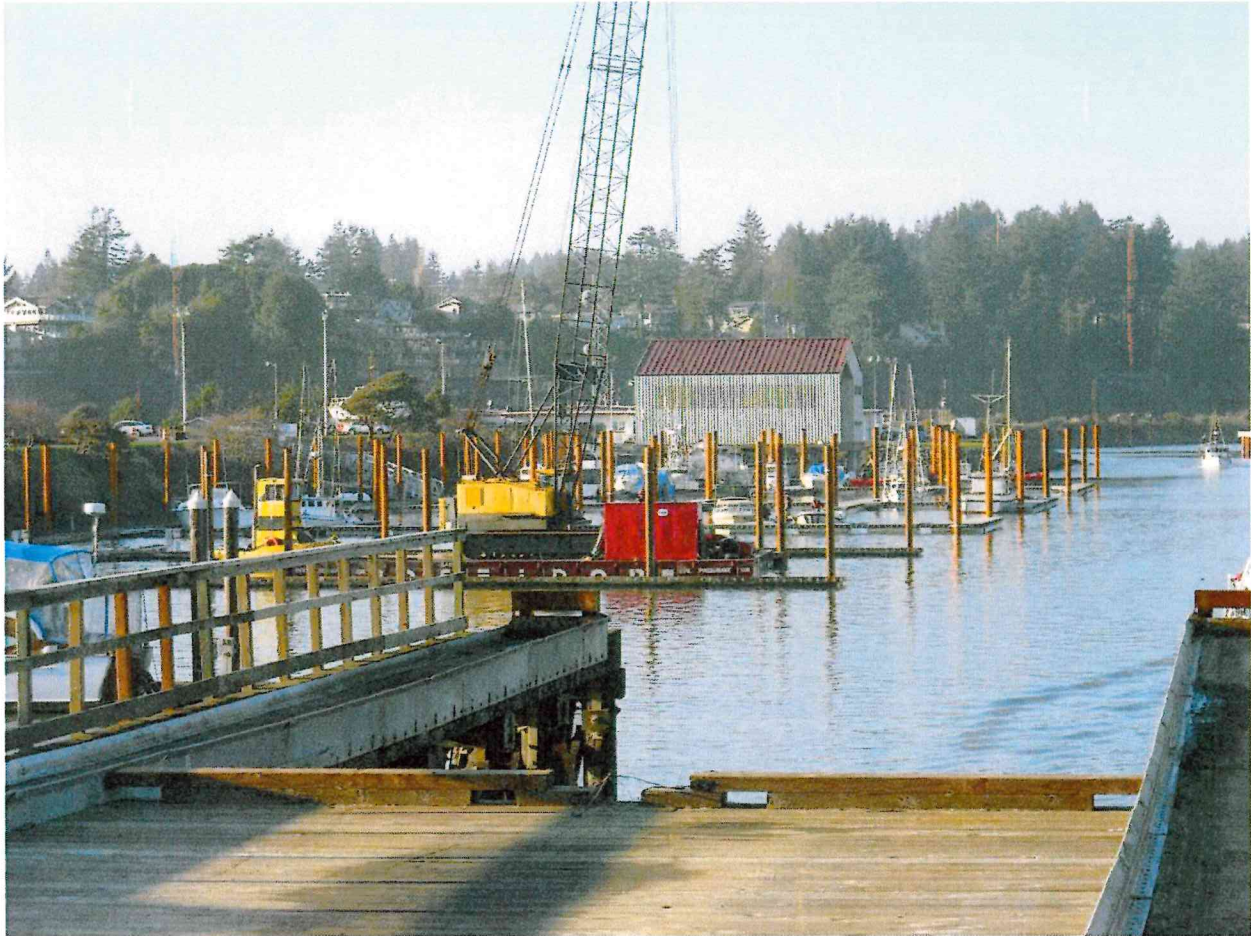
Port of Brookings Floating Dock Replacement
