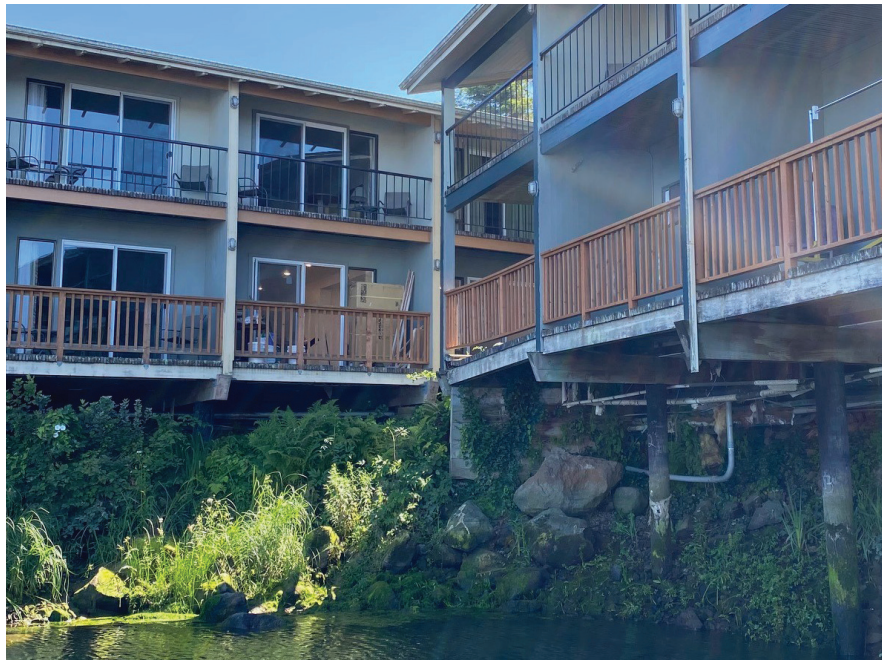
Figure 10: Chinook Building (above) and Astoria Riverwalk Inn (below)
